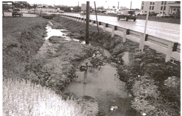
A municipal storm sewer outfall enters a stream that shows signs of contaminants.
