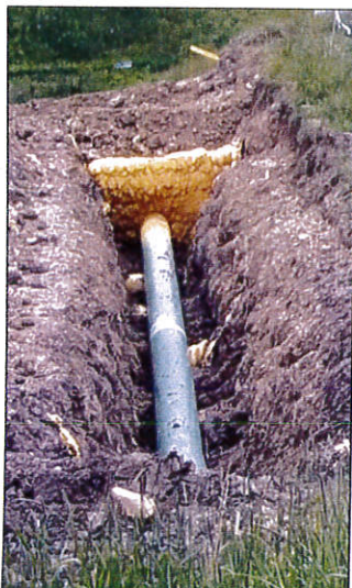
STANDARD CONSTRUCTION DETAIL # 13-4 Typical Trench Plug Installation
