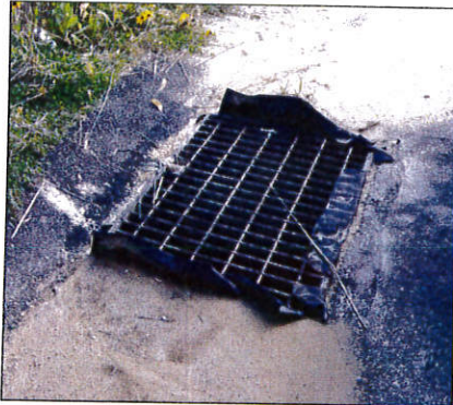
STANDARD CONSTRUCTION DETAIL # 4-16 Filter Bag Inlet Protection - Type M Inlet
